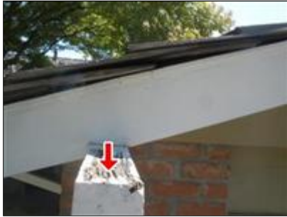
2.4 Picture 1 (Front decorative beam)
