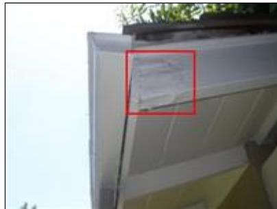
Item 5 - Picture 4 (Left rear barge rafter)
