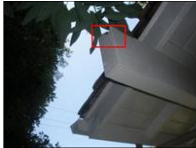
Item 5 - Picture 2 (Left rear decorative beam)
