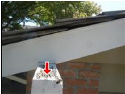
Item 5 - Picture 1 (Front decorative beam)
