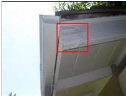
2.4 Picture 4 (Left rear barge rafter)
