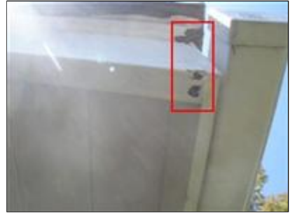
2.4 Picture 3 (Front left barge rafter and eave board)
